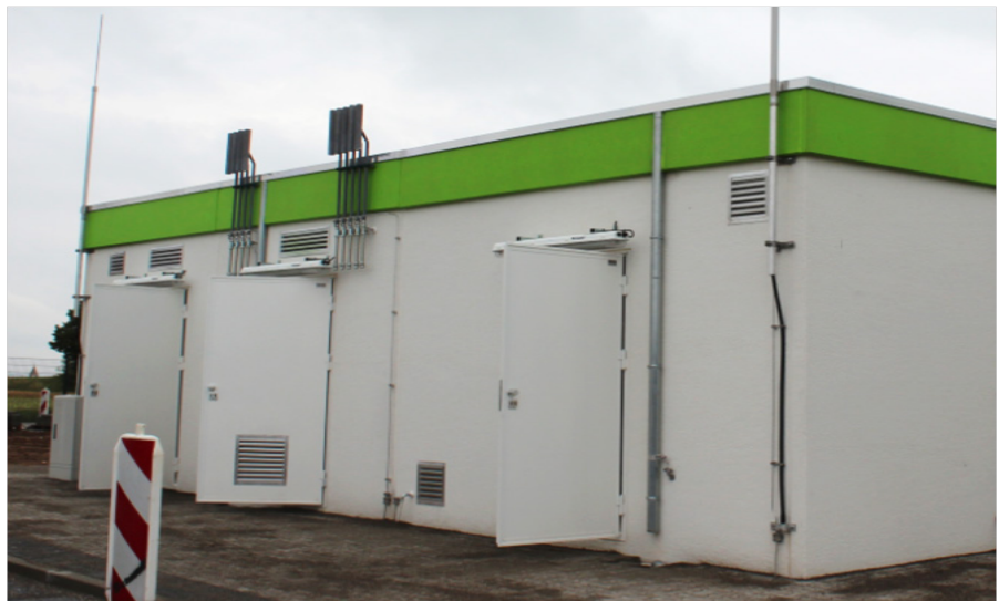
Abb. 7: Wall and pipe mounting: Internally routed isCon® down-conductor in interception rod in biogas plant
